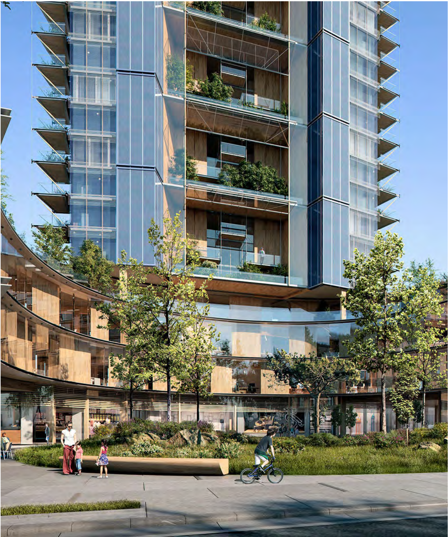
Figure 5.14: At 40 stories, Canada's Earth Tower will become the world's tallest hybrid wood tower, dramatically reducing the project's greenhouse gas emissions through carbon sequestration.
